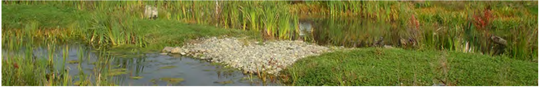
Storm-water management – storage
